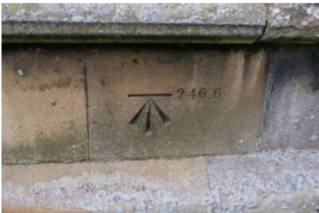
Figure 1: Typical Benchmark cut onto stone. This one has the height above sea level engraved with it.
